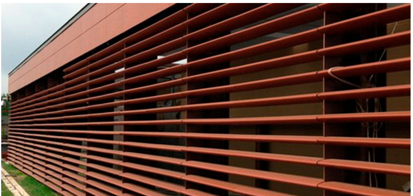
Project in Skolkovo, Russia.
