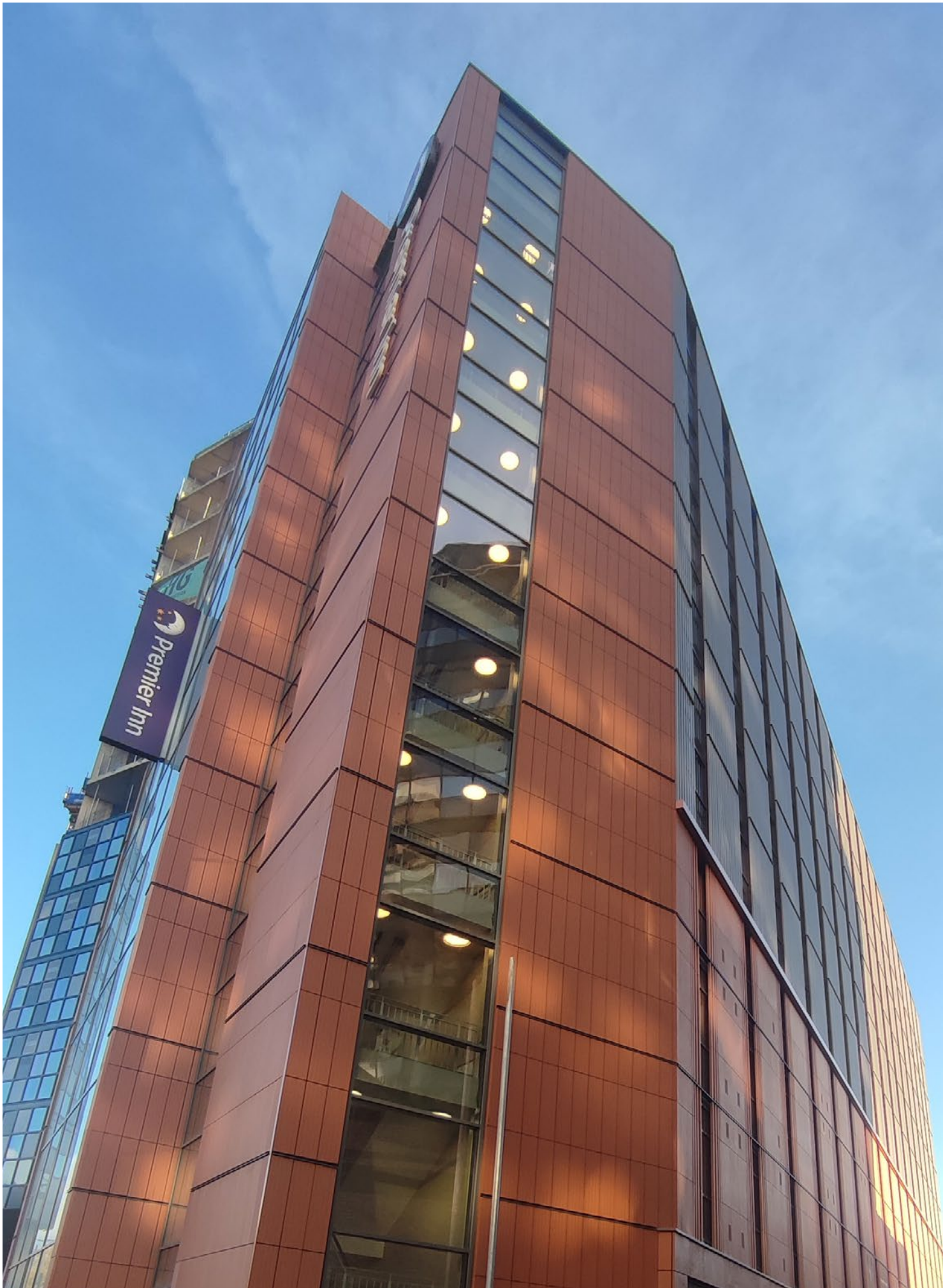
Hotel Premier Inn, Hammersmith, London, United Kingdom. Multifunctional UTM, square shutters and smooth panels of 1,200x600x40mm.
