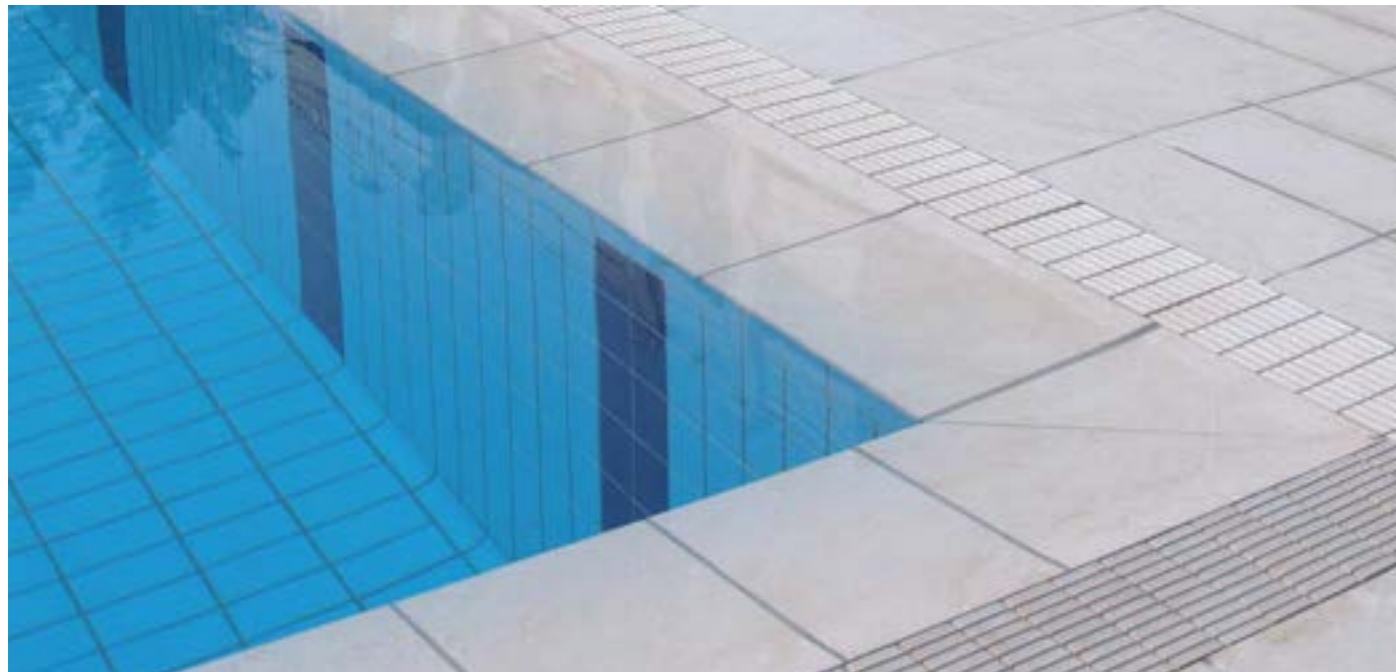
Rehabilitación de piscina comunitaria con borde 500 Beige Stone. Resfurbishment of community pool with 500 Beige Stone border.
